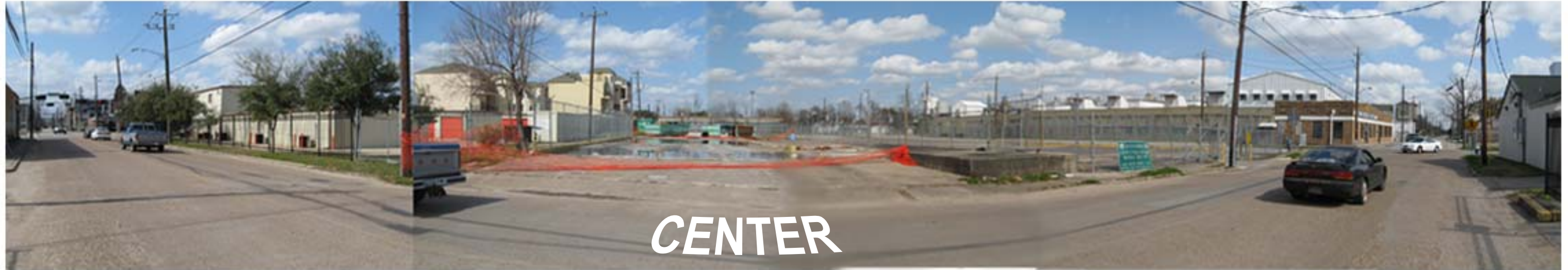
Panorama of Site View from Center St.
