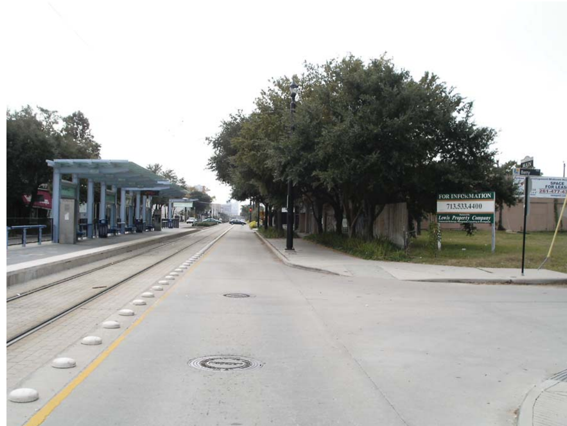
View South down Main Street
