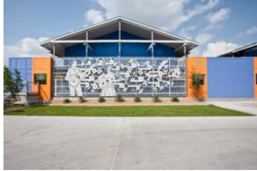
Category: Renovation/Restoration Glassman Shoemake Maldonado Architects, Inc New Hope Housing at Brays Crossing
