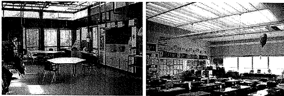
Figure 6: Seattle Classrooms With Clerestory Windows (left) and Central Skylight and Diffusing Louvers (right)
